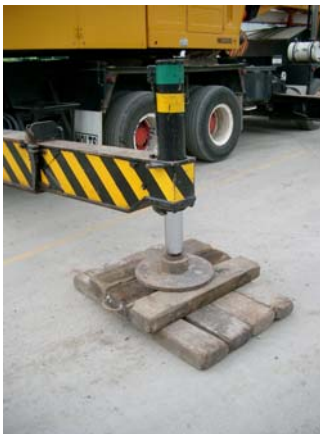
Figure 3 - Crane outrigger foot on timbers
