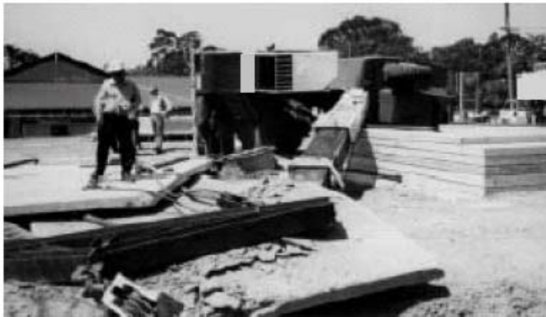
Diagram 7 – Rubber tyred pick and carry crane overturned
