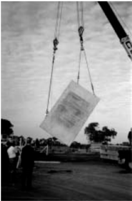
Diagram 11 – Rotation of a pre-cast panel
