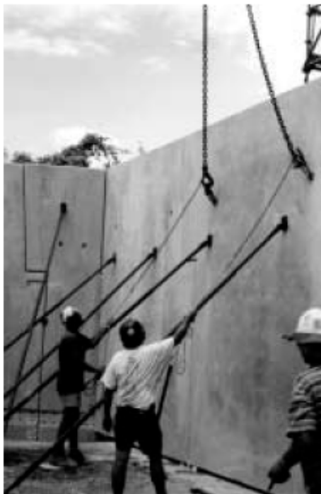
Diagram 9 – Lifting clutch release lines
